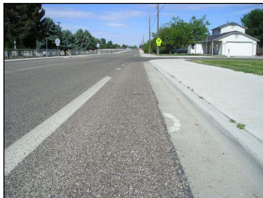
Boise Street bike lane stencil covered by chip seal and not re-stenciled
