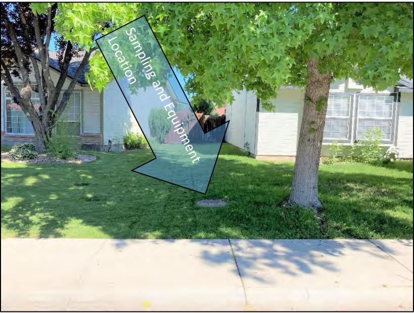
Station setting looking northwest – equipment in manhole
