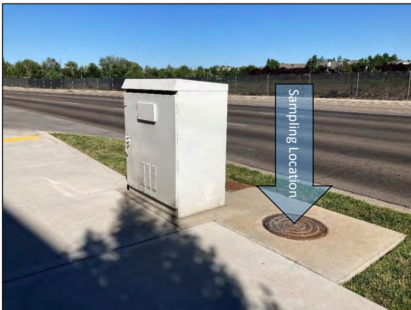
Station setting looking northwest
